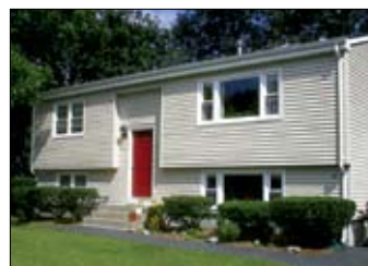
Haswill Street, Warwick
