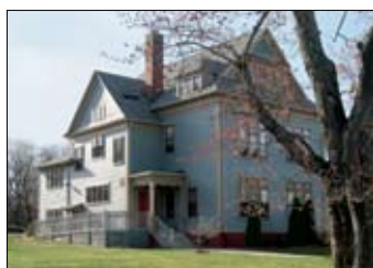
School House Place, Warwick
