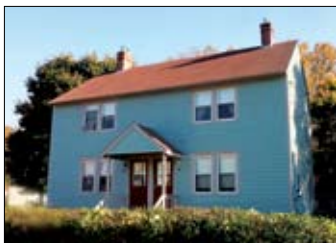
Bowling Lane, Westerly
