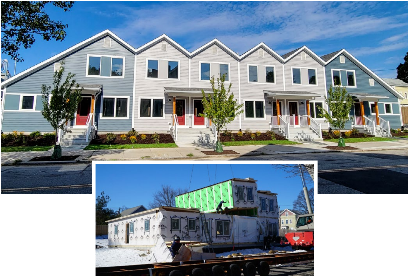
Bowdoin Street Rowhouse | One Neighborhood Builders | Providence, RI | 2022 | Modular Construction | Affordable Multifamily 20
