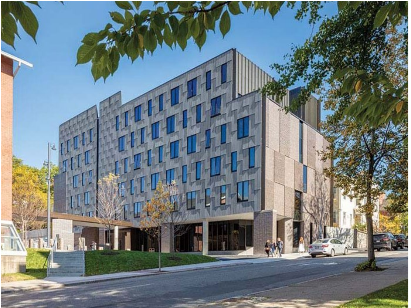
RISD North Hall | NADAAA | 2019 | Cross-Laminated Timber (CLT) Structure, Steel Frame
